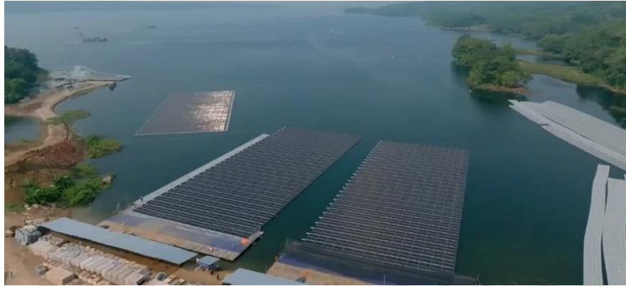
Fig. 3 A 145-megawatt floating solar plant
